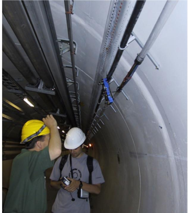
**Figure 1. Duct hanging in tunnel of CERN, span 1.5 m. Here the (microduct) cable blowing record of that time of 3.6 km was reached.**
