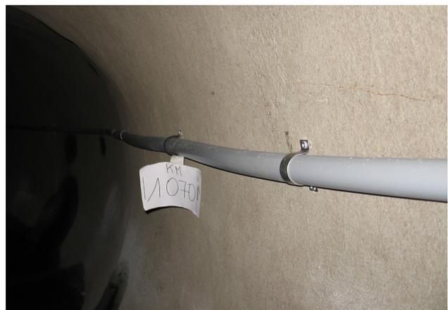
**Figure 2. Duct hanging in tunnel in Zurich (Switzerland), span 1.5 m. Here the cable floating record of 12.4 km was reached. The cable came out with 50 m/min.**
