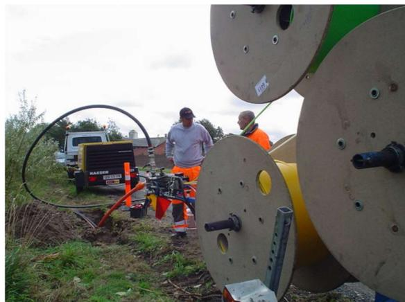
Fig. 13 Blowing loose bundle of microducts into a larger duct
