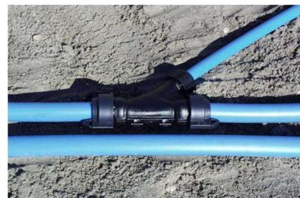
Fig. 15 Y-connector for branches in microduct networks
