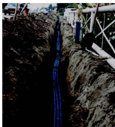
Fig. 3 Open trench with undulating ducts
