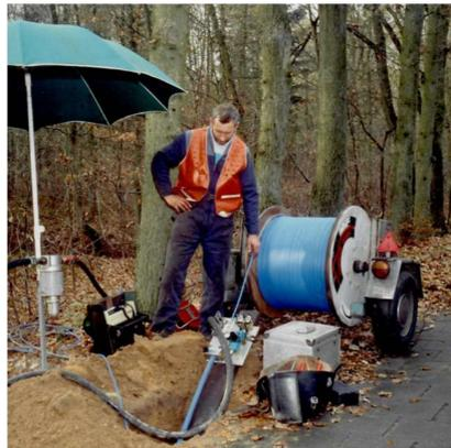
Fig. 8 First prototype of cable blowing machine in operation
