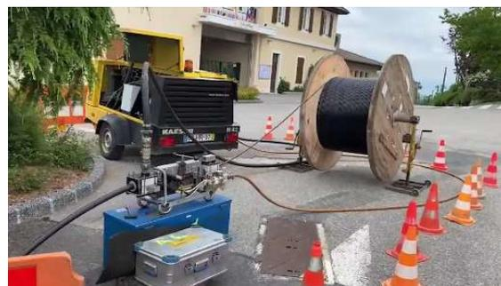
Fig. 10 Another commercial cable blowing machine in operation
