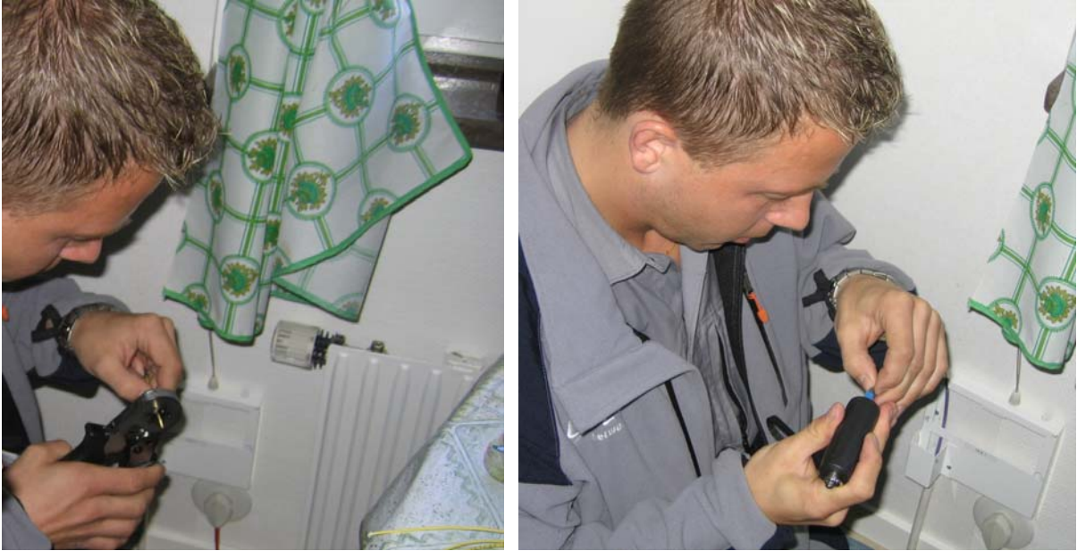
Figure 8: Crimping cylinder on ferrule (left). Pushing ferrule into connector housing (right)
