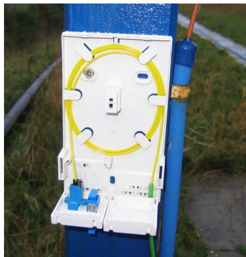
Figure 3: End of the IEC trajectory with Y-connector and termination box (left), latter close-up (right).
