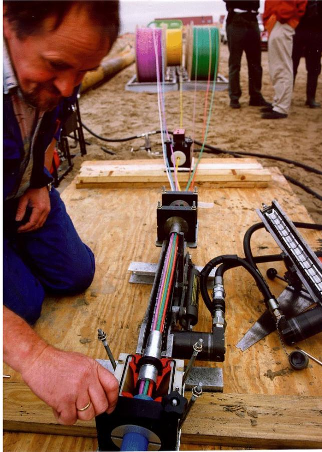
**Figure 2** Installation of a bundle of guide-tubes in a protective HDPE duct by blowing
