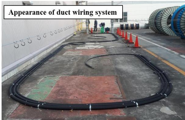
**Figure 8. Scheme of cable installation test**
