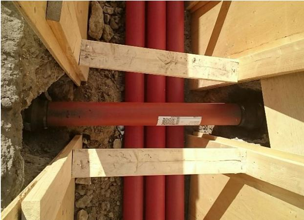
**Fig. 14: Problematic installation when crossing existing infrastructure which occupies the same depth as the cable system.**
