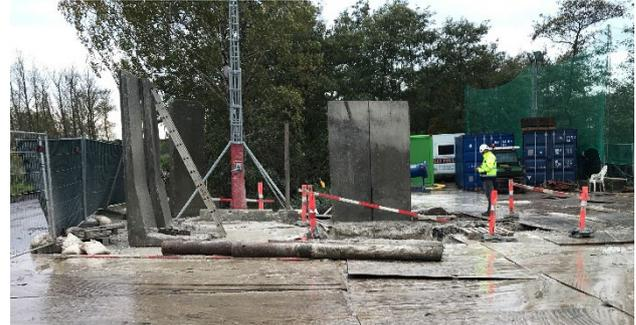
**Fig. 11: Protection from UXOs when performing HDD drillings in an old military shooting range.**
