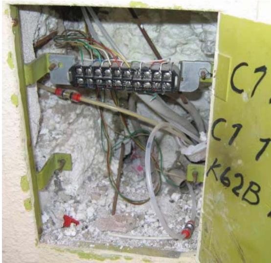
**Figure 14. Existing wall boxes with lack of space and microduct bend radius of 35 mm**
