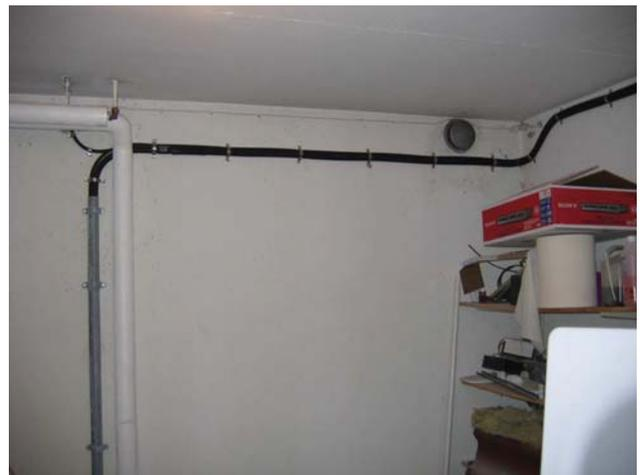
Figure 13. Bends in the bundles of 4/3 mm microducts, 12 of them in a black flame retardant flexible duct
