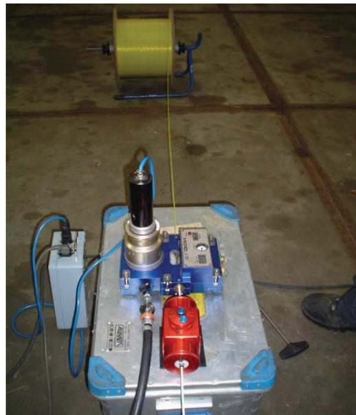
Figure 5. Blowing the preferrulized cable into a 4/3 mm microduct using blowing and lubricator unit
