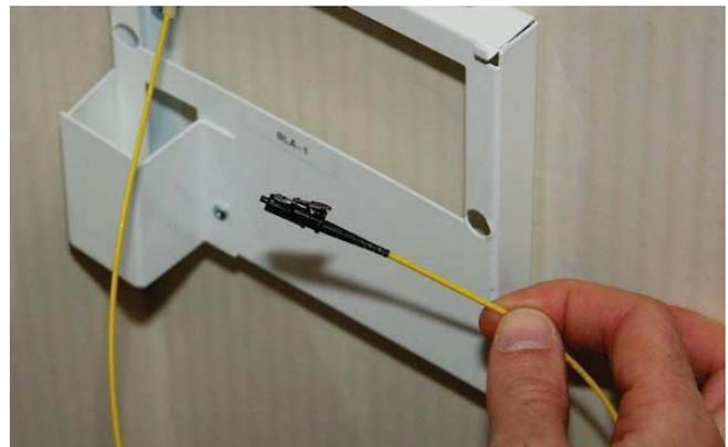
Figure 20. Finished connector
