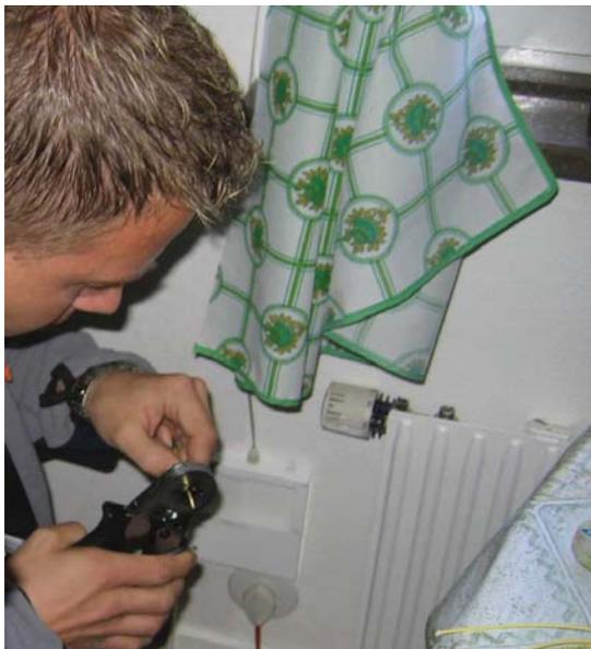
Figure 18. Crimping cylinder around ferrule holder
