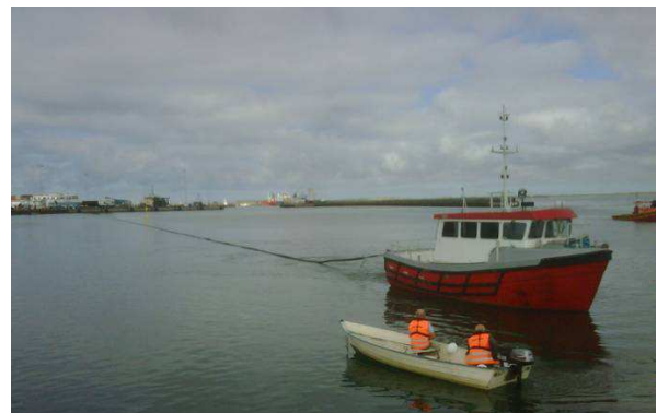
Fig. 13: Sailing out the pipe from the Jumbo drum
