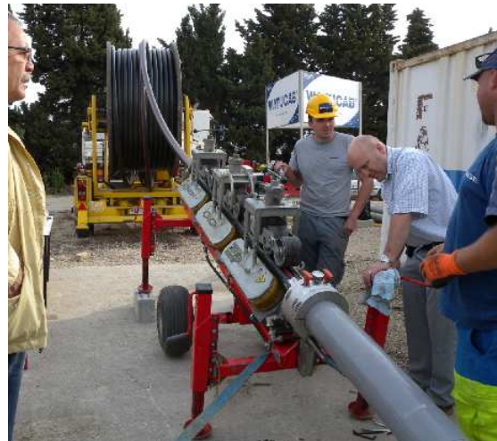
Fig. 4: Cable installed by water push-pull
