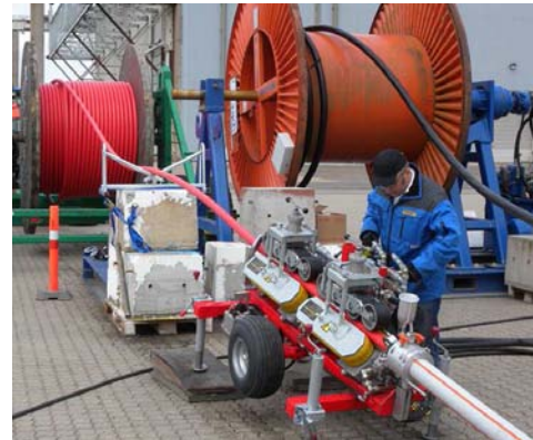
Fig. 7: Cables installed in Lindø trial
