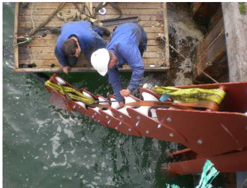
Fig. 14: Installation of pipe in bend restrictors
