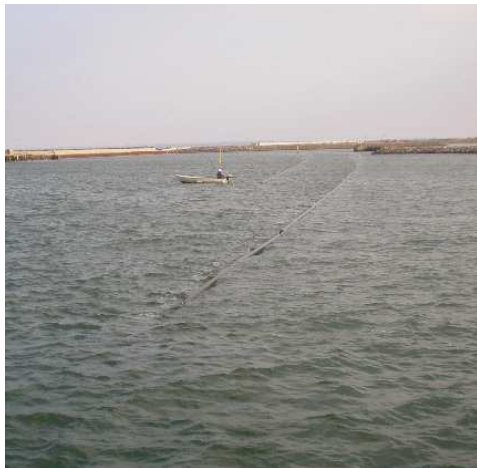
Fig. 15: Pipe sinking
