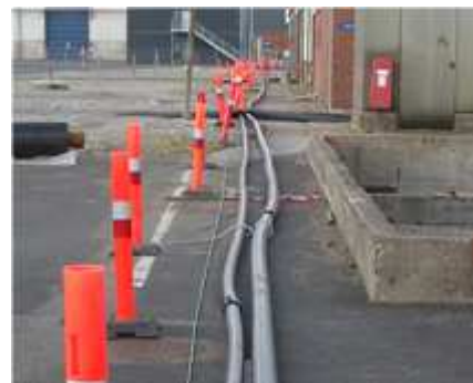
Fig. 8: Pipe couplings (every 100 m) in Lindø trial
