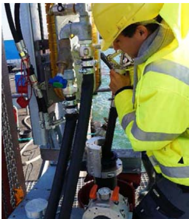
Fig. 16: Inserting Intelligent Pig
