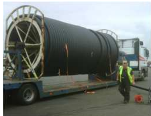
Fig. 12: Pipe supply on Jumbo drum
